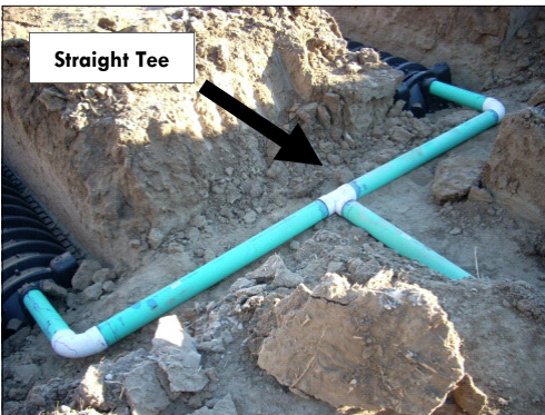
Straight tees (left) and four-way tees are not recommended because they will not evenly divide effluent entering the leachfield.
